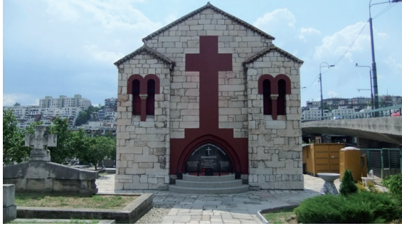
Plate 10: Orthodox chapel in Koševo cemetery, Sarajevo, designed by Belgrade architect Aleksandar Deroko, with graves of Heroes of St. Vitus, and memorial plaque dated 28 June 1939, (Photo SH, 5 July 2013)
